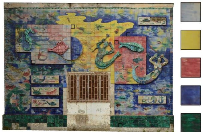
*Fig. 2. Colourimetric features. On the left, the orthophoto of the façade, obtained by digital photogrammetry. On the right, the main color tones used within the composition.*
