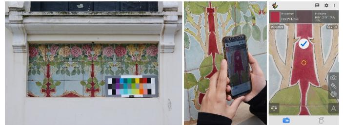
Fig. 7. The colour acquisition phase: on the left, the majolica band photographed with the colour checker; on the right, the experimentation carried out with the smartphone application.
