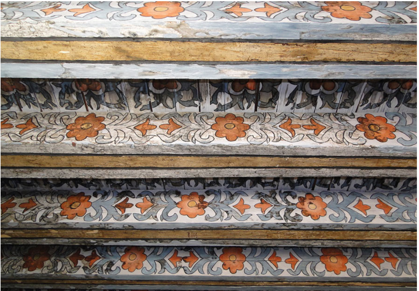
Fig. 8 View of the beams after the color correction. Note that the same blue hue was used for the chromatic reintegration, despite the difference in the hue of the original paint (Photo: Muñoz-Alcocer, K., 2024).
