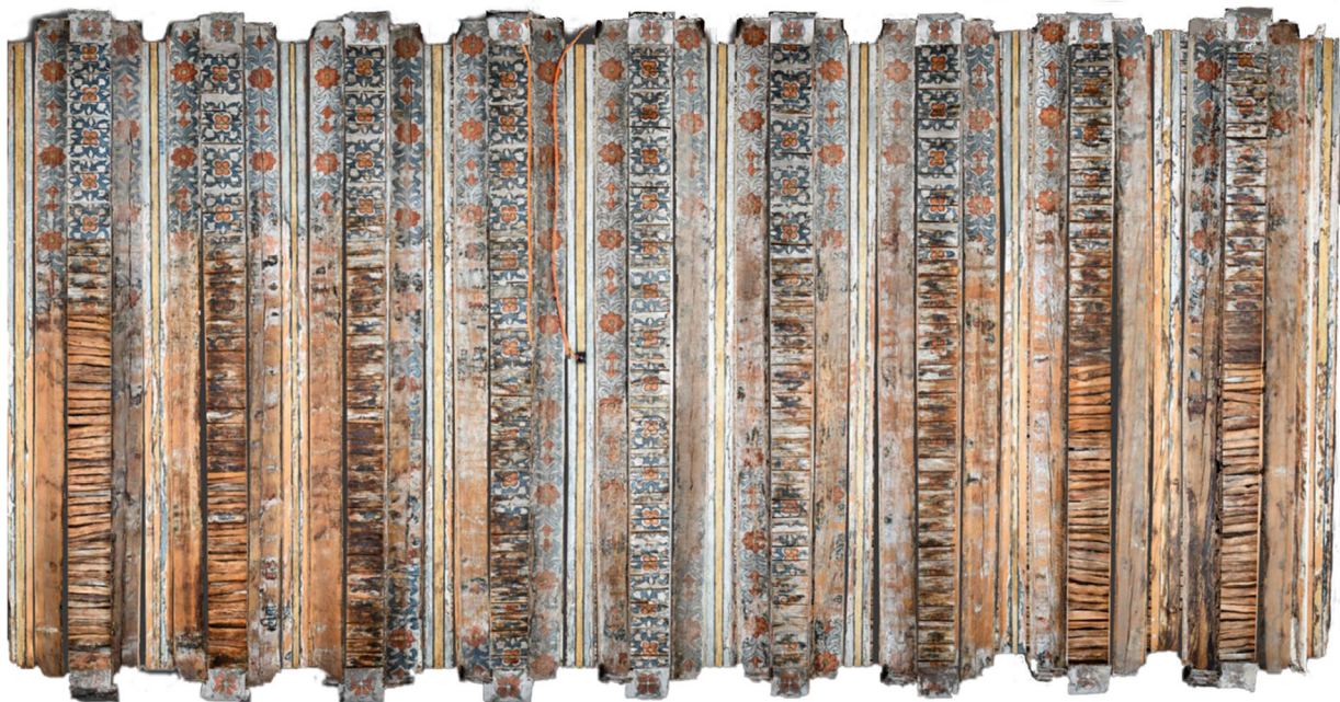
Fig. 5. Photogrammetry image of the ceiling before the intervention. It is possible to observe the three face-sides of the beams. Note the blue color tone variations between the beams, including at beam-face that is not exposed to light. (Photogrammetry & imaging: Misiones Coloniales de Chihuahua A.C., Montes Treviso F., 2024).
