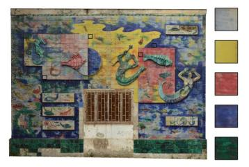
Fig. 2. Colourimetric features. On the left, the orthophoto of the façade, obtained by digital photogrammetry. On the right, the main color tones used within the composition.
