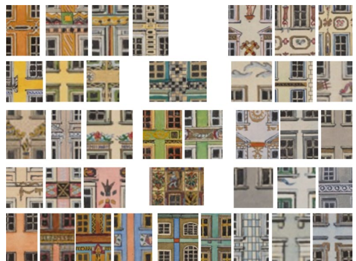
Fig. 2. Details of all the building façades above the ground floor level facing the Market Square from the 1928 colour design proposal.
