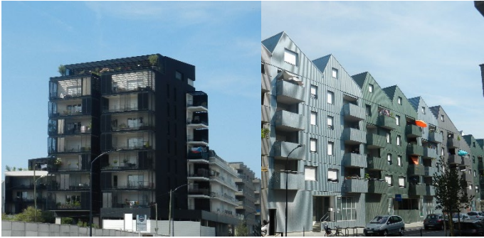
Fig. 3. The Bassins à Flot district: two apartment buildings. Photos © A. Herbert.
